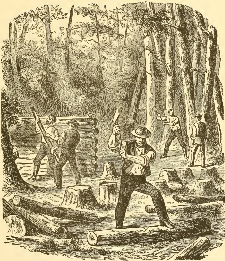
BUILDING THE FIRST HOUSE AT JAMESTOWN.
